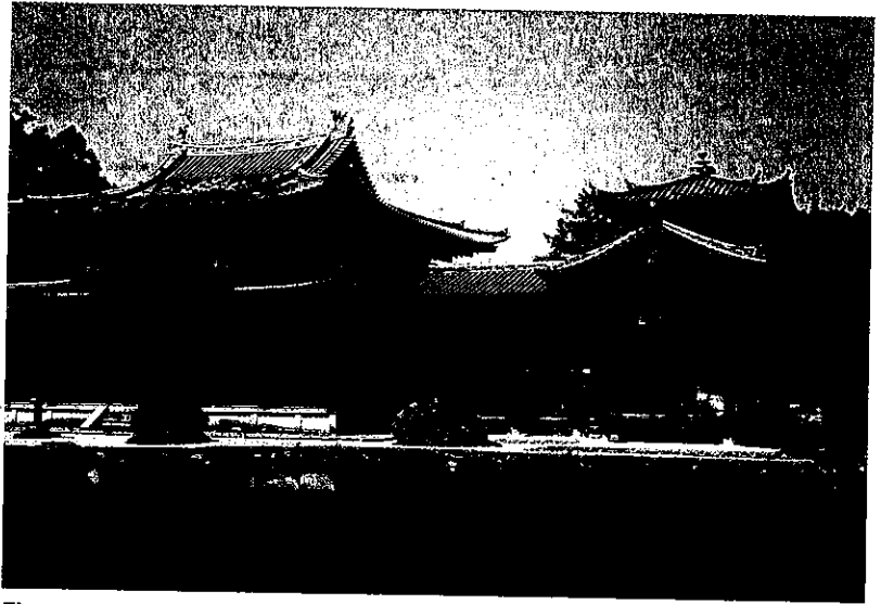
Figure 12.3 Tang era architecture at the Phoenix Pavilion in Japan. Some of the most characteristic features of this splendid style of construction are its steeply sloping tiled roofs with upturned corners, the extensive use of fine wood in the floors, walls, and ceilings, and the sliding panels that covered doors and windows in inclement weather and opened up the temples or monasteries to the natural world on pleasant days.
